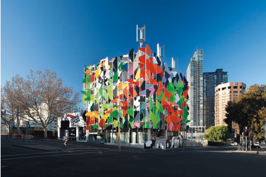
Fig. 3.11 Pixel Building, Melbourne. Grocon's Pixel building is the first carbon neutral office building of its type in Australia (Courtesy studio505, Dylan Brady & Dirk Zimmermann. Melbourne, Australia / photo: John Gollings)
